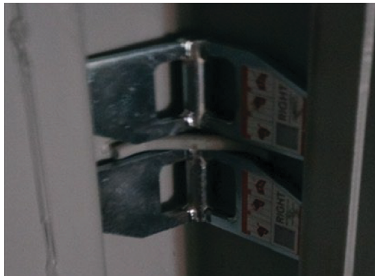
Figure 6.2.11 - 2 Method 6.2.11 - CornerLash® anchors installed
